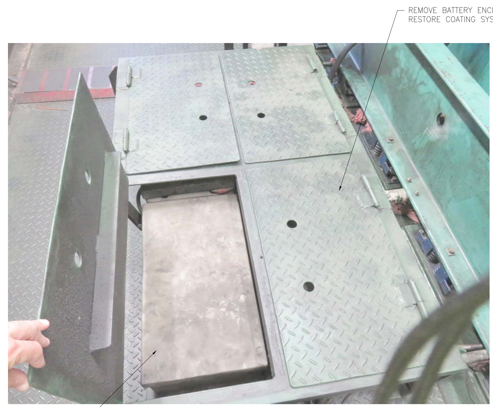
ITEM "D" - REMOVE BATTERIES AND ENCLOSURE
