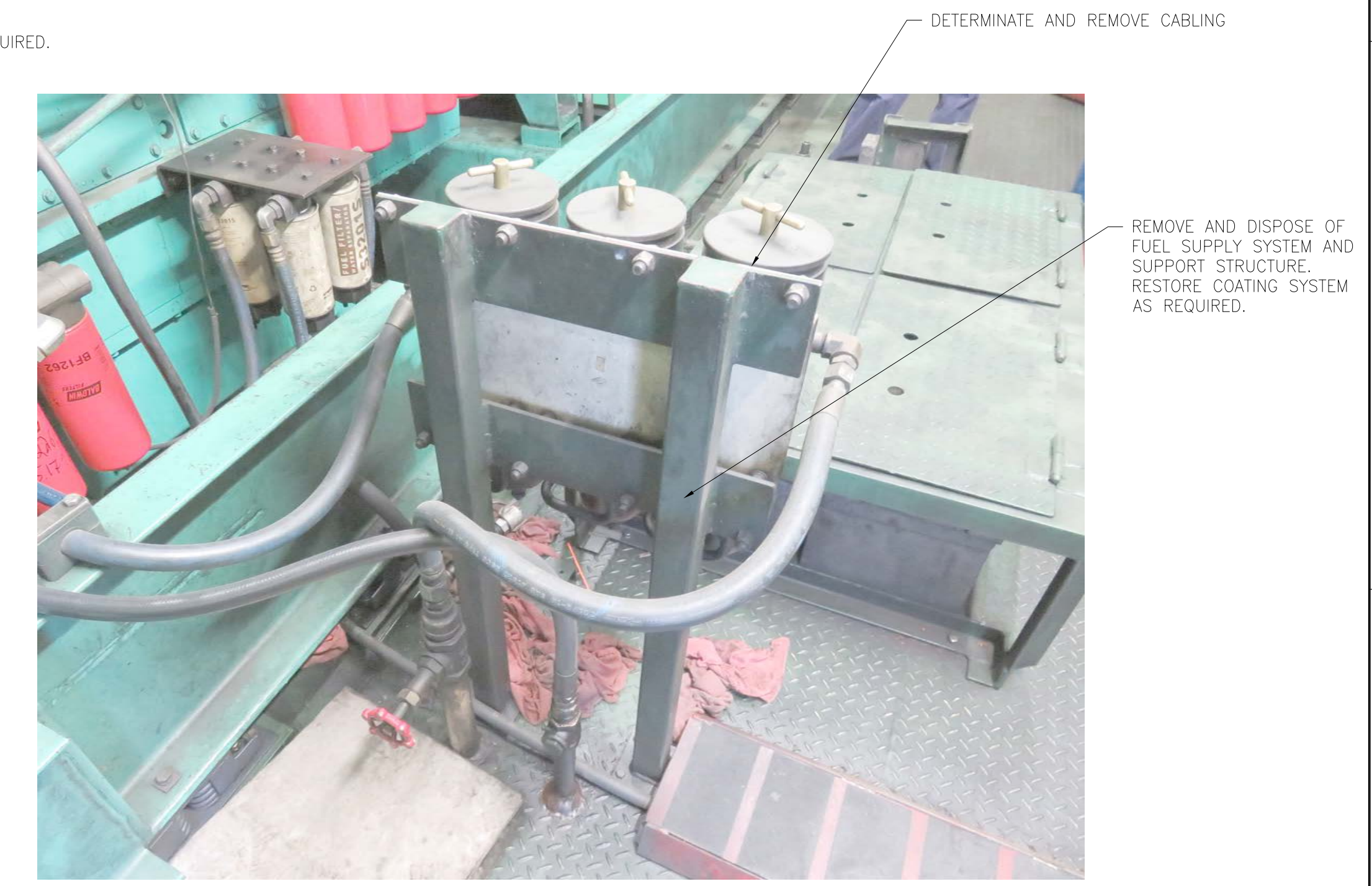
ITEM "E" - REMOVE FUEL SUPPLY SYSTEM
