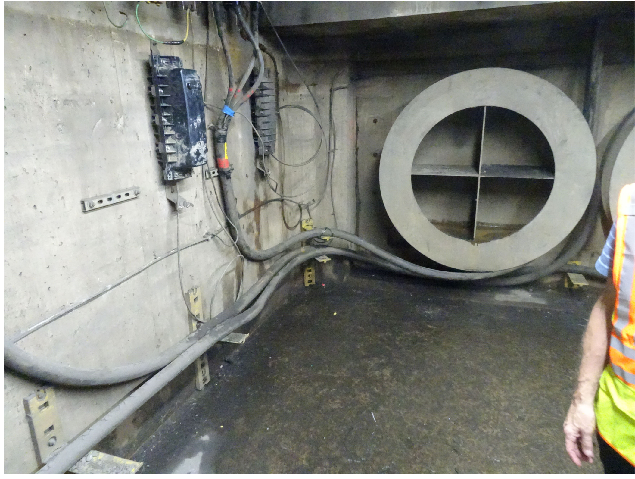
STS PIT NO. 2
