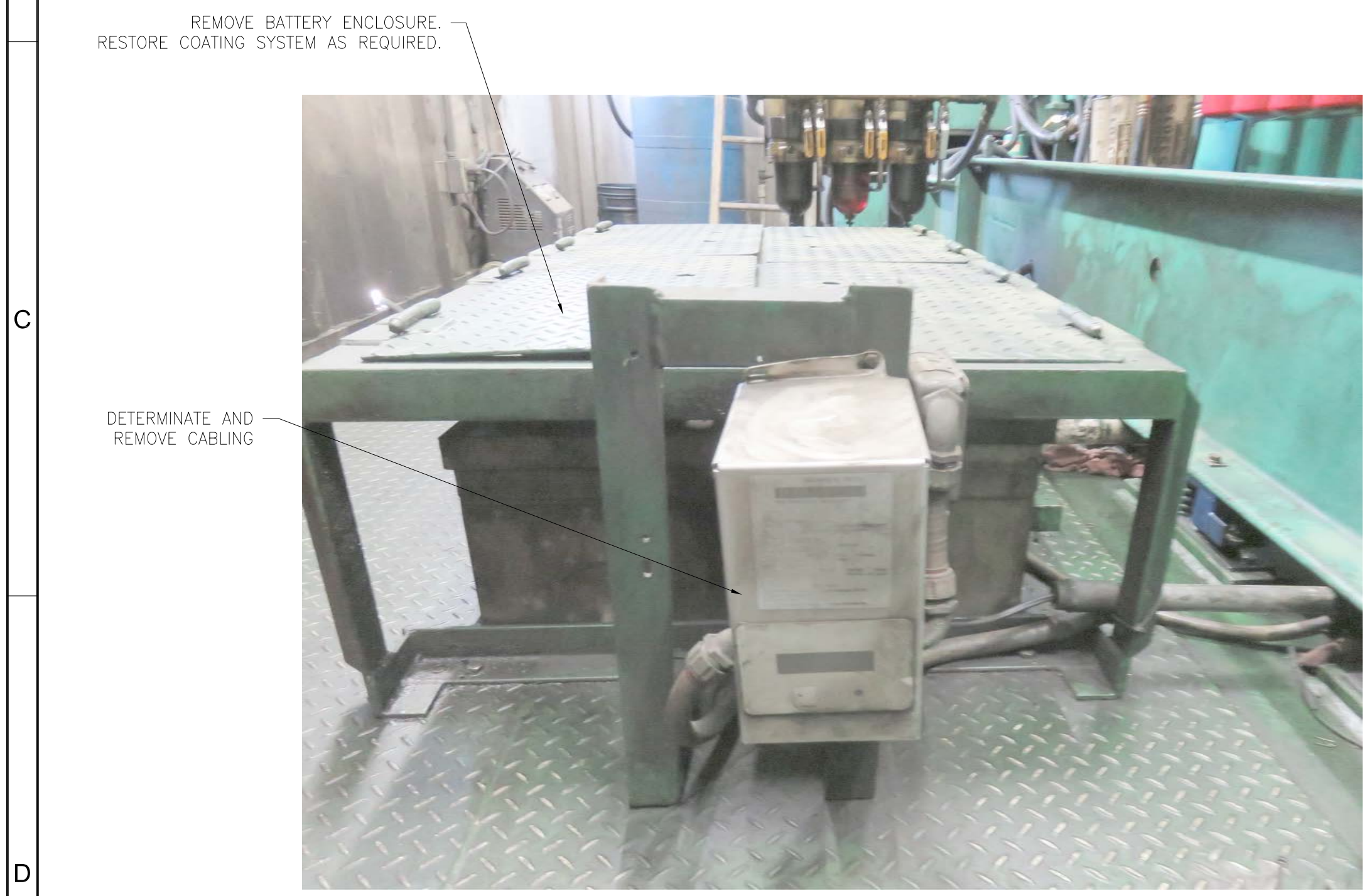
ITEM "D" - REMOVE BATTERIES AND ENCLOSURE
