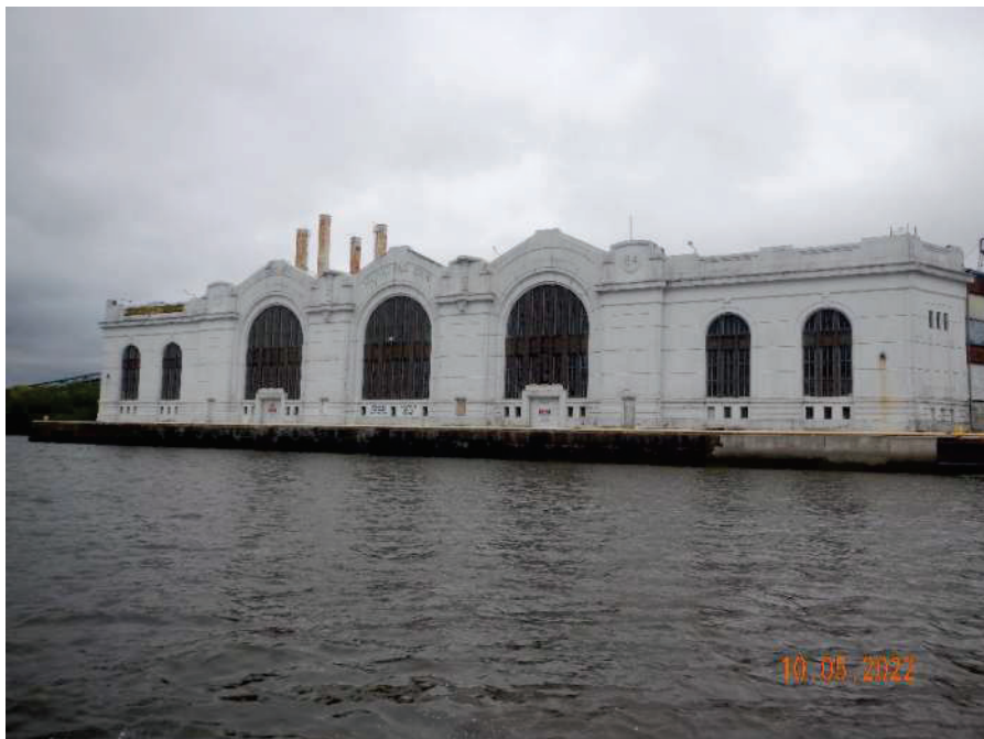
Photo 4: East Elevation of the Pier 84S Warehouse
