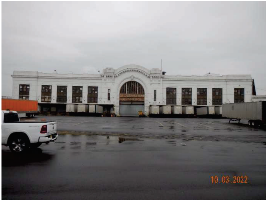
Photo 3: West Elevation of the Pier 84S Warehouse
