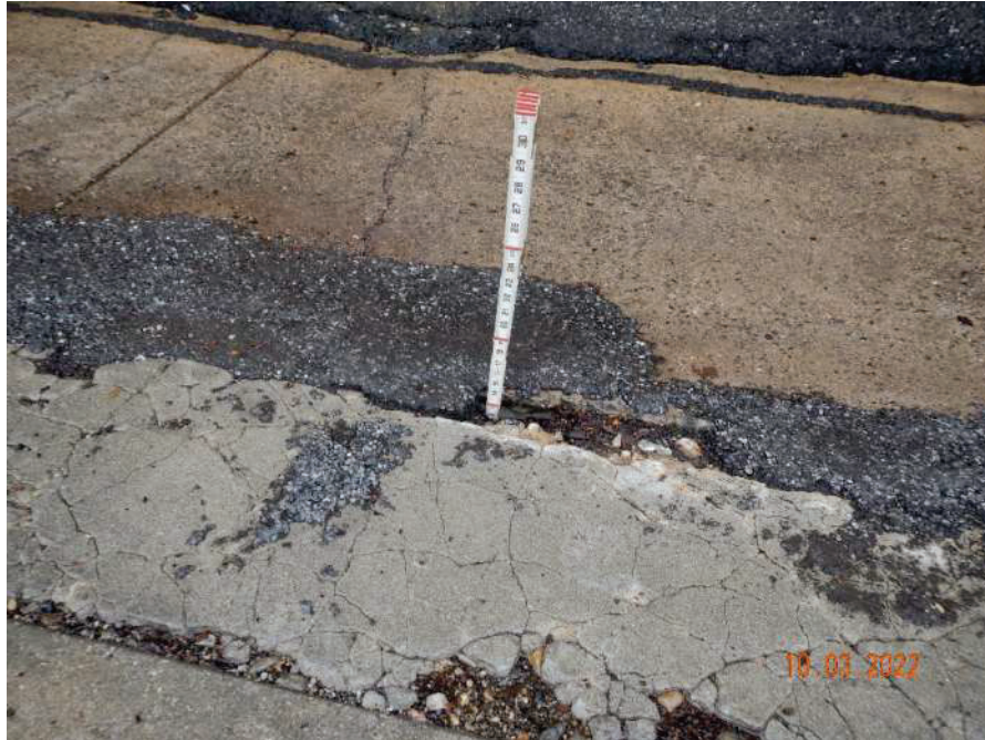
Photo 15: Area of separation between widened and original sections (North Apron shown)
