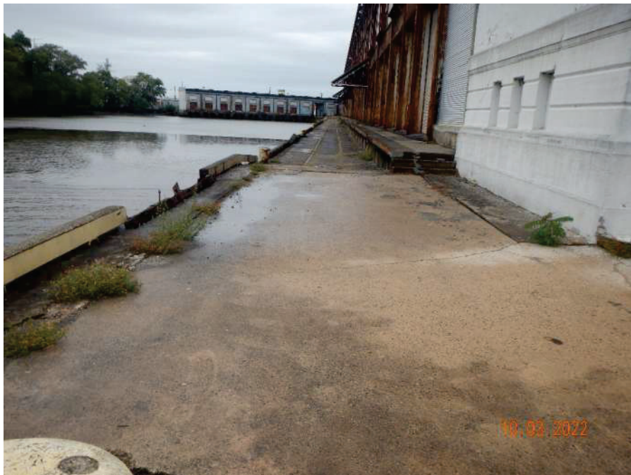
Photo 8: Typical view of South Apron Looking West
