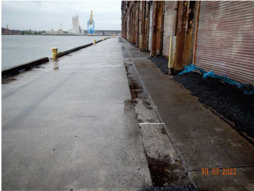
Photo 5: Typical view of North Apron Looking East
