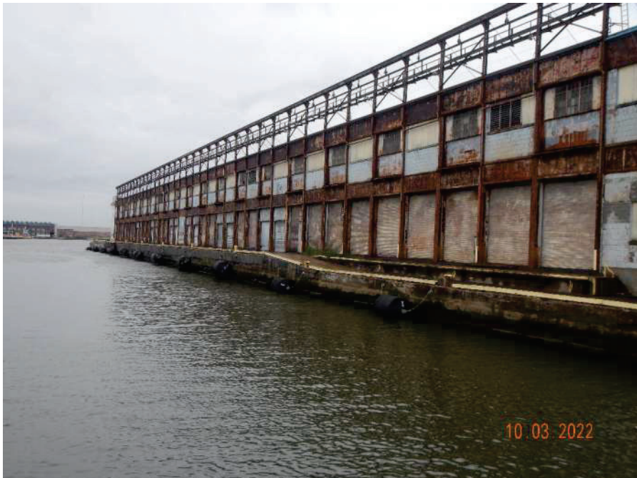
Photo 2: North Elevation Looking Southeast
