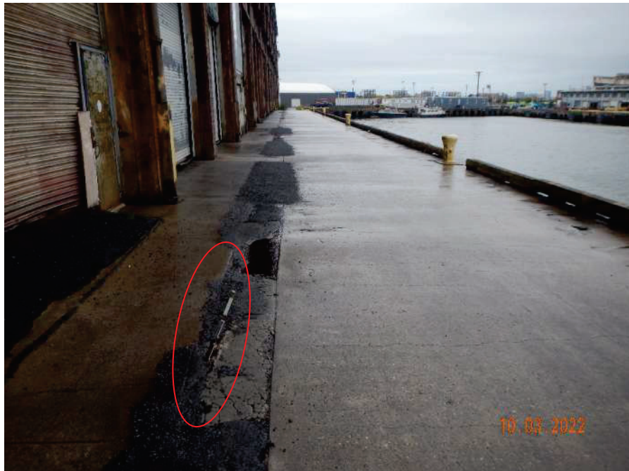
Photo 14: Area of separation between widened and original sections (North Apron shown)
