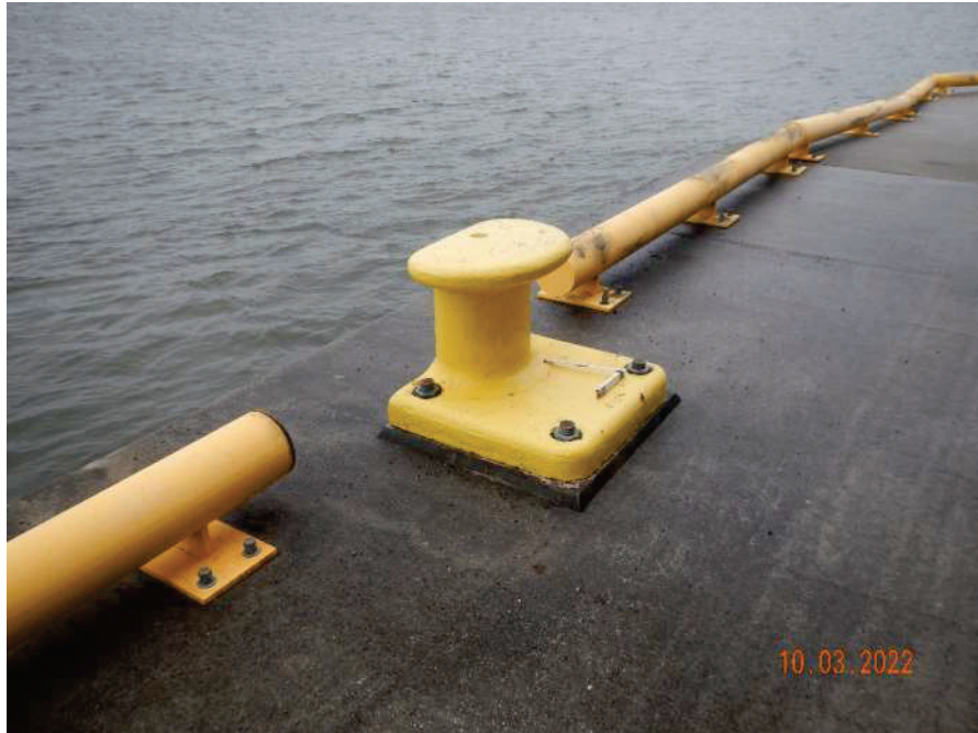
Photo 22: Replaced bollard at the Northeast corner
