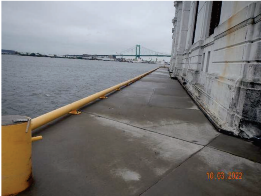
Photo 7: Typical Condition of East end
