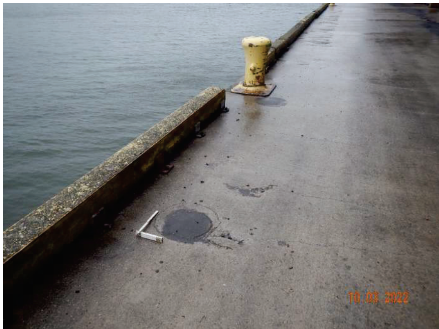
Photo 12: Typical Patch in top of deck for Aux. steel pipe pile
